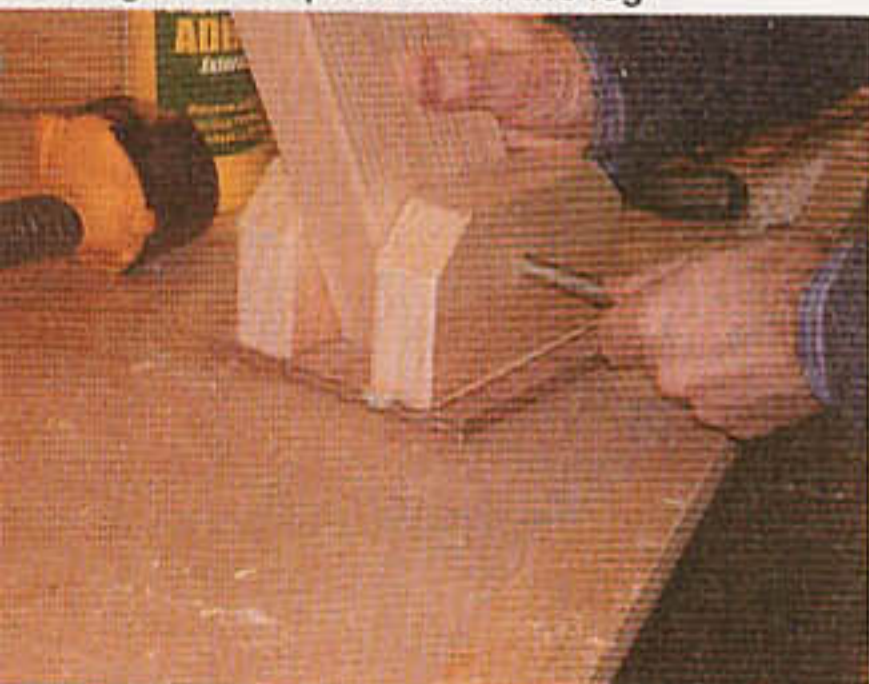
Marking the bolt position on the leg
